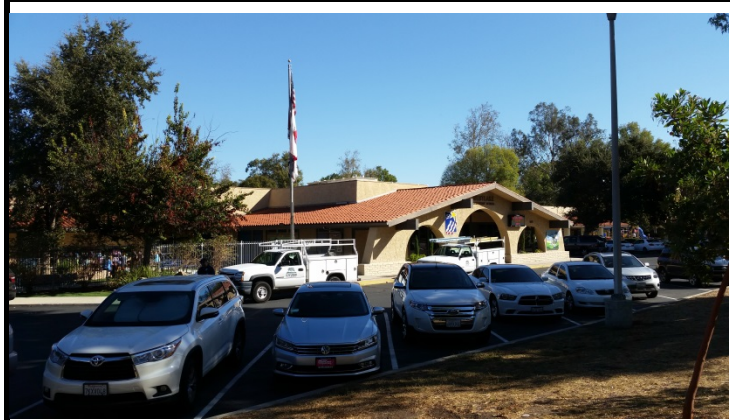
Photo 1 Building Name: Admin/Multi Purpose Building Building Number: 1 Description: View of main entry from parking lot.
