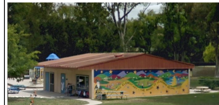
Photo 4 Building Name: Kindergarten Building Building Number: 4 Description: Kindergarten Building, currently used as a transitional kindergarten classroom.
