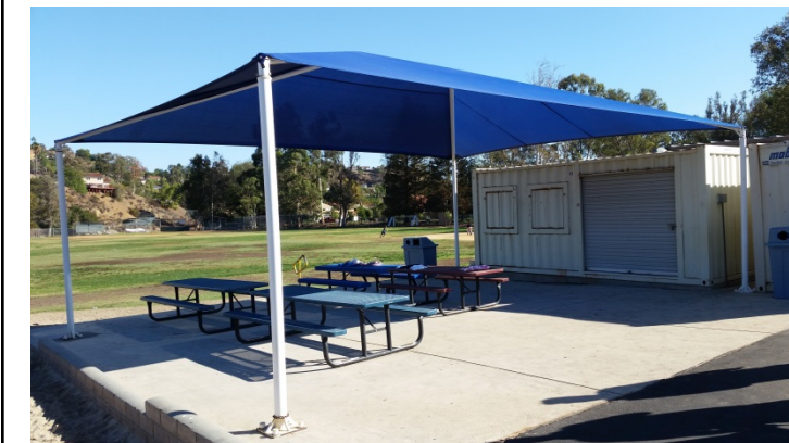
Photo 8 Building Name: Shade Structure Building Number: 9 Description: Lightweight steel structure with fabric canopy cover.
