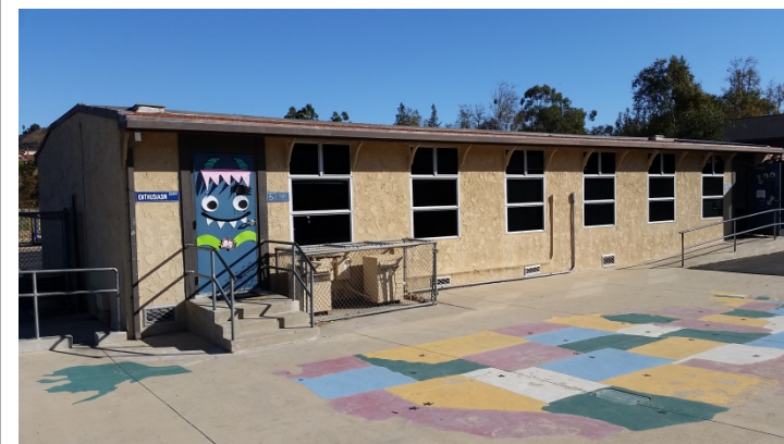
Photo 7 Building Name: Classroom Building Building Number: 8 Description: Two portable classrooms one of which is a maker space; the maker space classroom is only accessible through the use of stairs.
