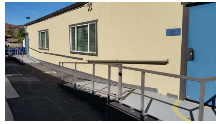
Photo 2 Ramp access to portable Classroom Building 5.
